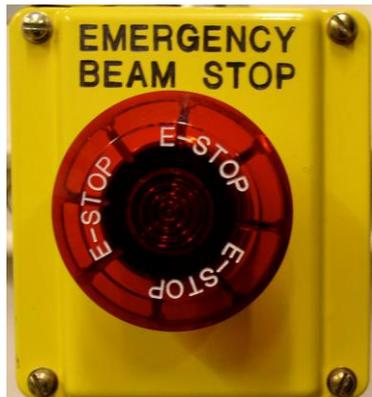
In the event that you become accidentally locked inside the experiment hutch, push the E-STOP button to prevent beam from entering the station. Then use the Emergency Door Release Mechanism to open the station door. Push the Auto Open button located on the panel. The door should automatically slide open. If this fails, press the Manual Open button and open the door by hand.
